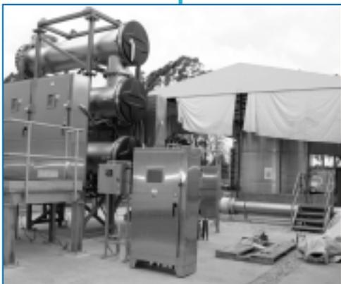
Construction of the Phox advanced oxidation ultraviolet (UV) system by Trojan Technologies began in summer 2003. The GWR System will contain nine UV Phox systems, and each system will treat up to 8.75 million gallons of wastewater per day. When complete, it will be the largest UV treatment system designed for NDMA removal in the world.
