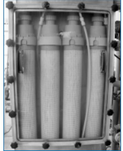
Here are four microfiltration modules used in the US Filter CMFS microfiltration system chosen for the GWR System. Each module contains 14,000 hollow fibers that reject anything over 0.2 micrometers in diameter. The GWR System will have a CMFS microfiltration system consisting of a total of over 15,000 membrane modules — the largest ever installed by US Filter.
